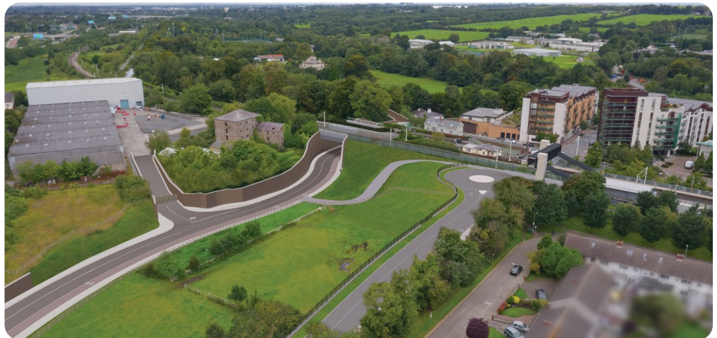
Aerial view of Level Crossing Replacement at Ashtown (Trees removed from image to provide improved view of accessibility bridge)
