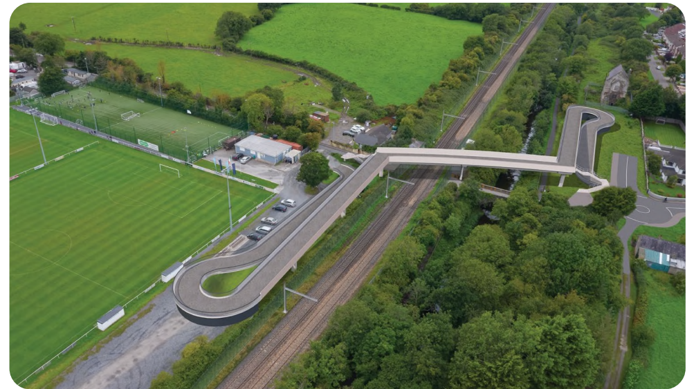
Aerial view of level crossing replacement at Porterstown
