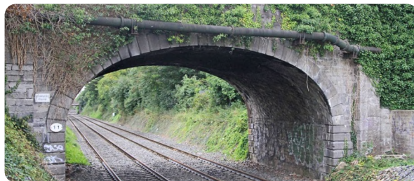
View of Castleknock Road Railway Bridge
