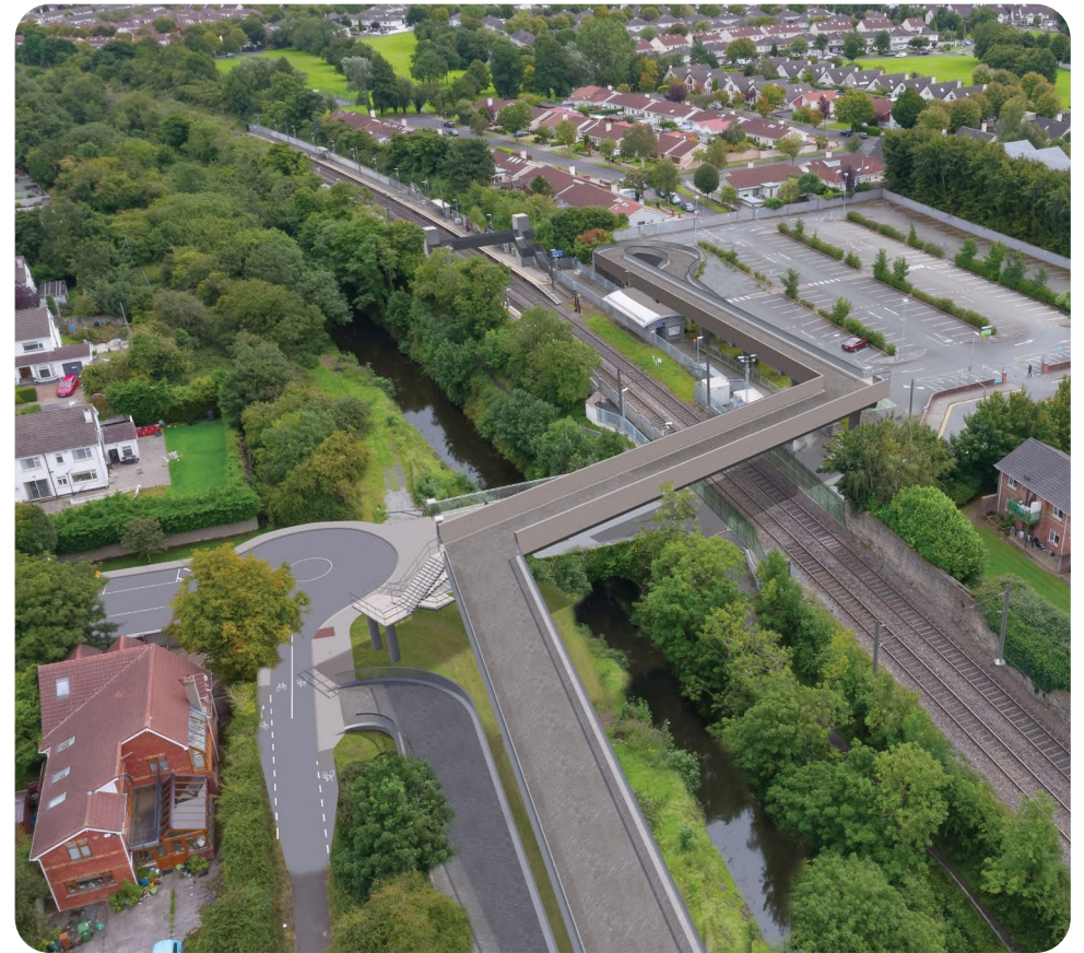
Aerial view of Pedestrian and Cyclist Bridge at Coolmine
