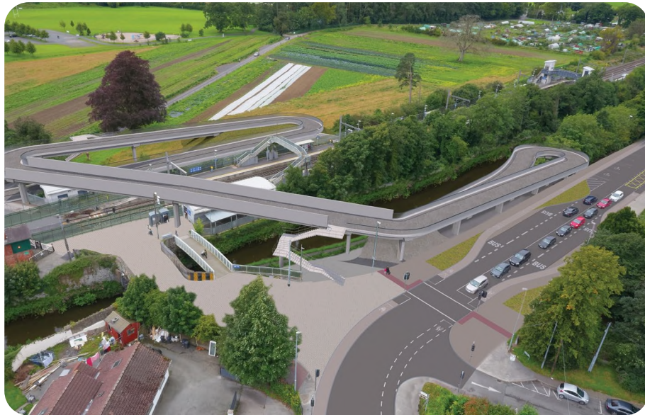
Aerial view of Level Crossing Replacement at Clonsilla
