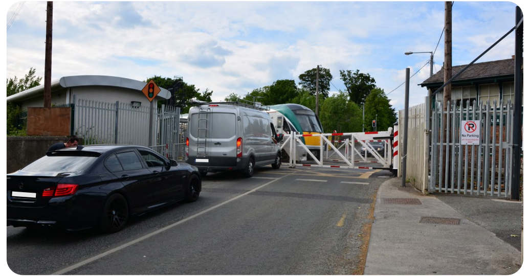
Image of Existing Clonsilla Level Crossing
