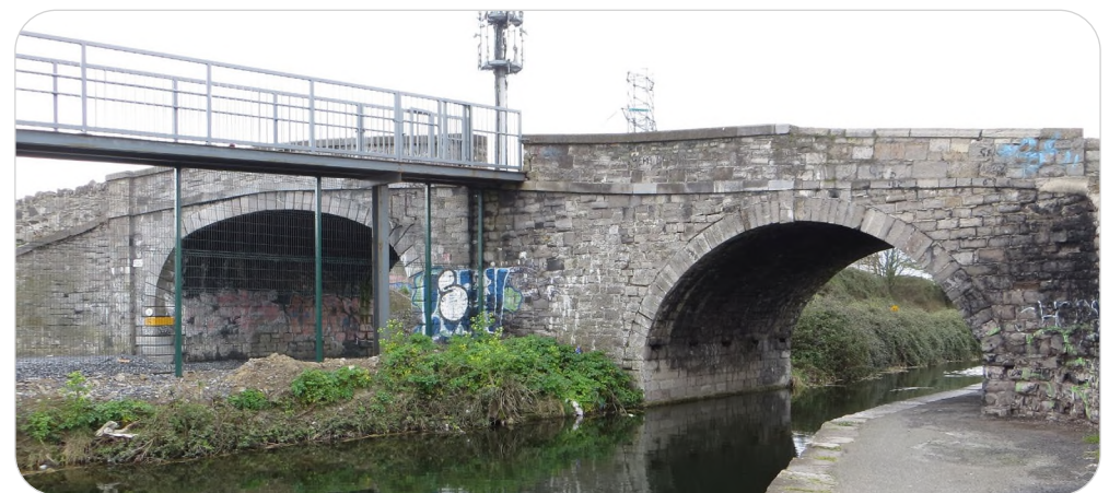
View of Broombridge (Canal and rail arches)
