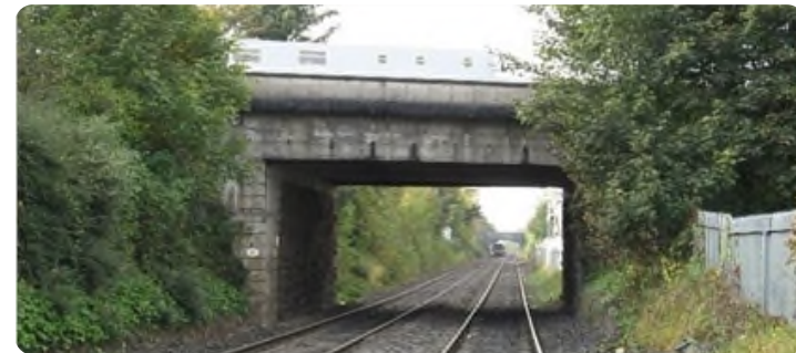
View of Old Navan Road bridge
